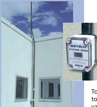
The ERITECH ERICORE Downconductor is easily retrofitted to existing structures. Inset: ERITECH® Lightning Event Counter (LEC IV) installed to register strikes to ERITECH® SYSTEM 3000.
